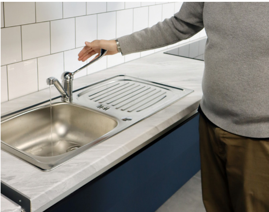
Above: Shallow sinks and lever taps with paddle lever handles aid those with limited mobility and dexterity
